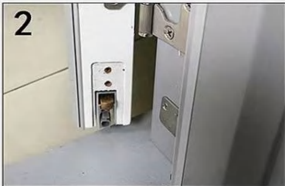
Rotation adjustment to close the door Seal to floor position
