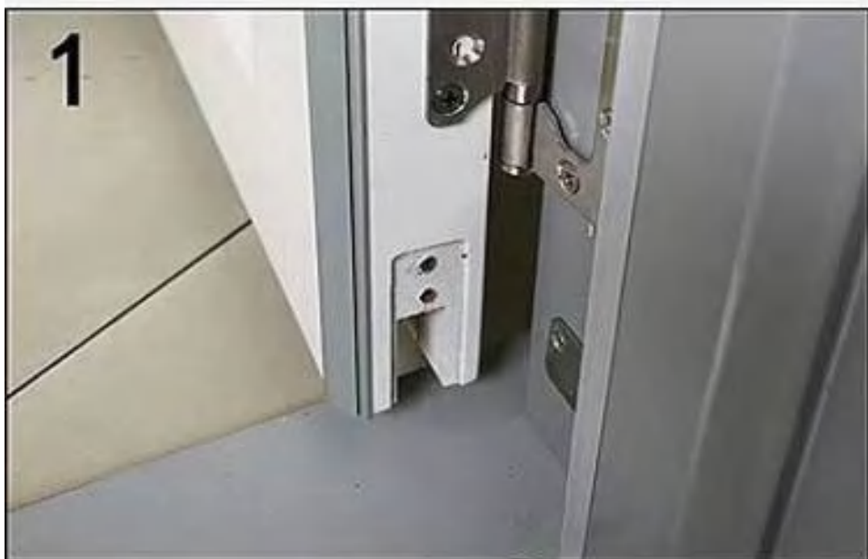
Rotation adjustment to close the door Seal to floor position
